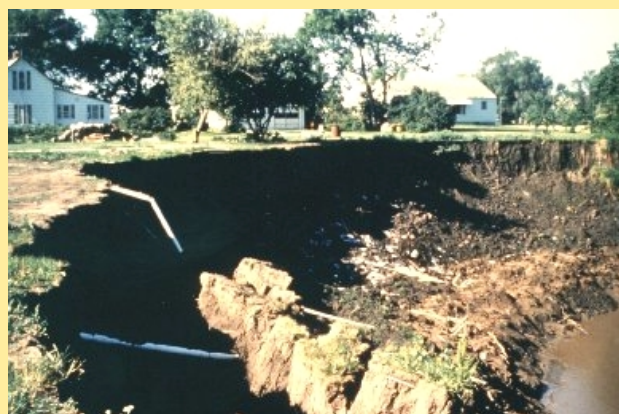
Fig. 1.1-1 Failed streambank threatens nearby homes.
