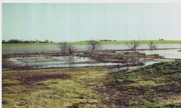
Fig 2.3-14 Floodplain diversion site Clarendon, TX
