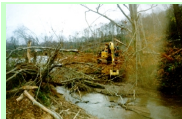
Fig. 2.3-2 Debris removal using heavy equipment (backhoe), Bethel Road site, Hall County, GA
