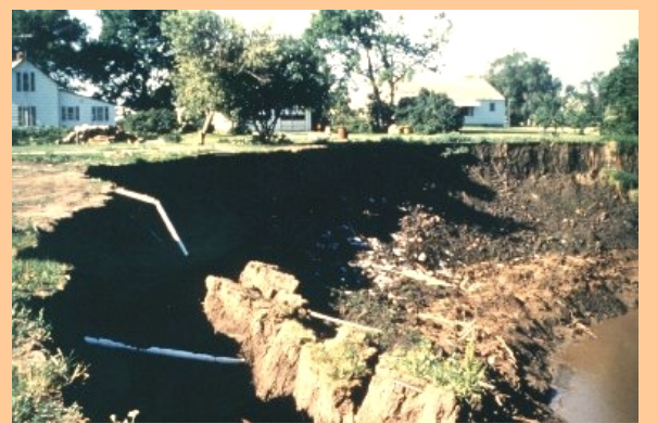
Fig. 2.3-4 Property threatened by a failed streambank
