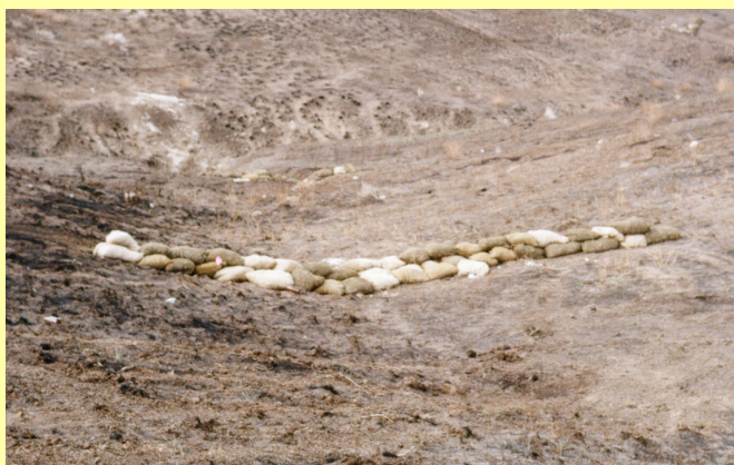
Fig. 2.3-19 Grade stabilization structure, 8th Street Burn, Boise Hills, ID
