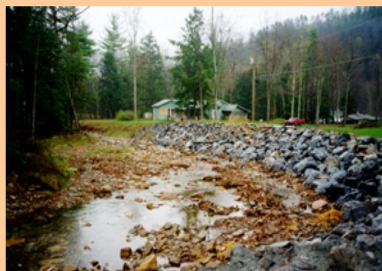
Fig. 2.3-6 Riprap installed at Rocky Run, VA
