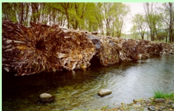
Fig. 2.3-7 Rootwads installed at Rose River, VA
