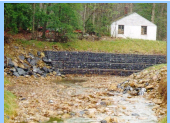
Fig. 2.3-5. Gabions installed at Rocky Run, VA
