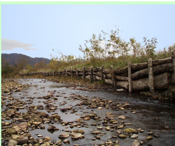
Fig. 2.3-8 Timber cribbing structure, Cherokee County, NC
