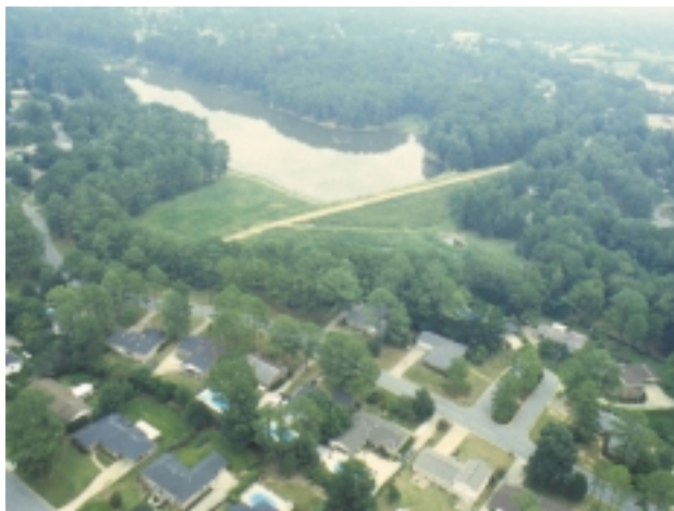
Figure 8 . . . Homes Built Downstream From a Dam Can Adversely Affect Public Safety
