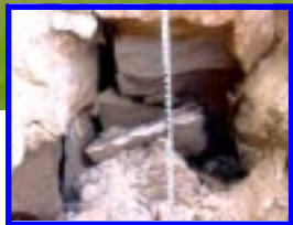
Seepage in the embankment has resulted in partial failure of the dam.
