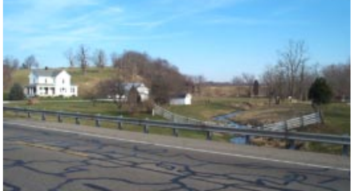
The dam protects a state highway and homes located 1300 feet downstream.
