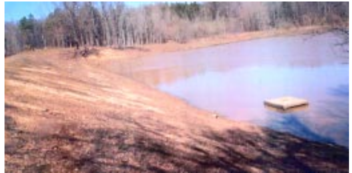
Dam Number Y-17-74 is one of three dams being rehabilitated.
