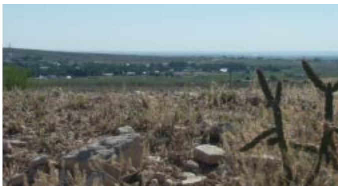
Hackberry Dam No. 2. View from auxiliary spillway showing protected area and homes downstream.
