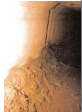
THE PROBLEMS. Top: Dam blowout of Coon Creek #41. Bottom left: Freeze-thaw damage to the concrete cradle which supports the pipe. Joint separation can be seen at the top of the photo. This is at Plum Creek #19 in Pierce County. Bottom right: At Alma Mill Creek Structure #2 in Buffalo County, soil from the dam has collapsed through the gap in the pipe. The weakened dam is more vulnerable to failure in heavy rains.
