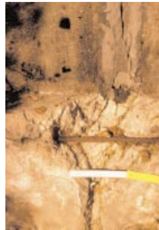
THE PROBLEMS. Top: Dam blowout of Coon Creek #41. Bottom left: Freeze-thaw damage to the concrete cradle which supports the pipe. Joint separation can be seen at the top of the photo. This is at Plum Creek #19 in Pierce County. Bottom right: At Alma Mill Creek Structure #2 in Buffalo County, soil from the dam has collapsed through the gap in the pipe. The weakened dam is more vulnerable to failure in heavy rains.
