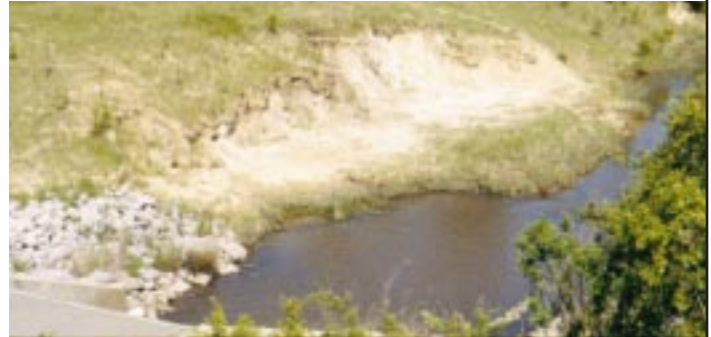
THE PROBLEMS. Erosion on a spillway is the culprit, above, while debris causes problems with an outlet pipe, left, at a Lee County site. These and other problems must be corrected to ensure the dams continue to provide flood control.
