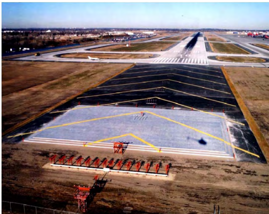
FIG AD 1.1-51 Engineered Materials Arresting System (EMAS)
