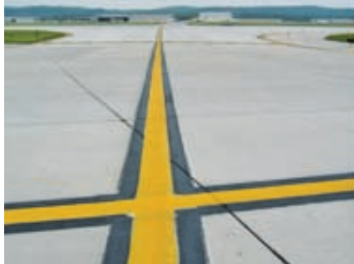
Figure 14 Enhanced Taxiway Centerline Markings
