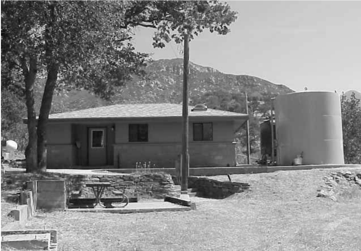
FIGURE 7. WATER TREATMENT SYSTEM BUILDING
