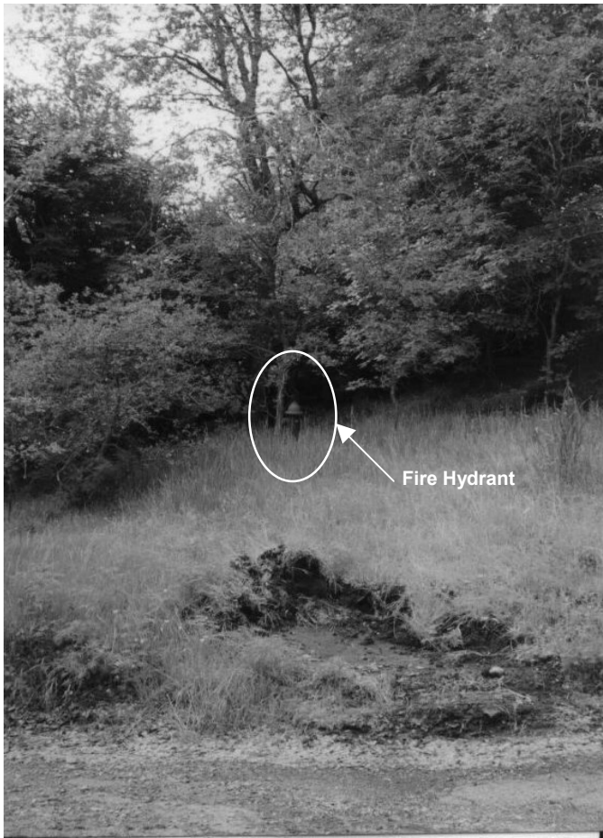
FIGURE 4. INACCESSIBLE FIRE HYDRANT
