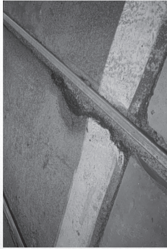
Figure 16-12. POTENTIAL PROBLEM: Broken surfaces should be avoided at railroad crossings. A surface material that will not buckle, expand, or contract significantly should be used near railroad tracks.
