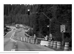
As part of ODOT's efforts to maintain mobility and provide sustainability, a solar powered traffic signal was used to control traffic at the Odell Creek Bridge site on Oregon 58.
