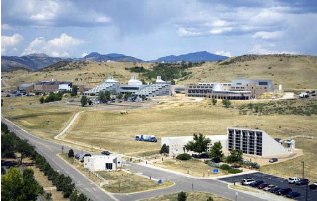
The Laboratory's permanent site near South Table Mountain will soon expand with the addition of an administrative support building, wood-fired boiler plant and more.
