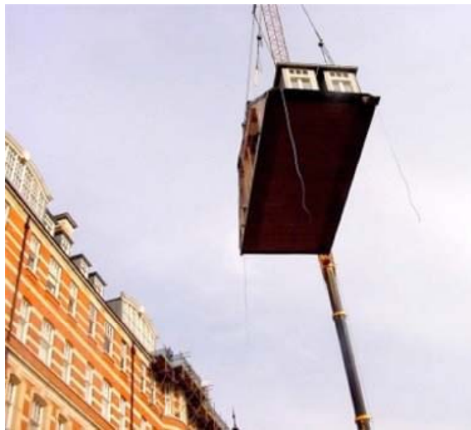
Figure 2 Modular penthouse being lifted into position atop an existing building
