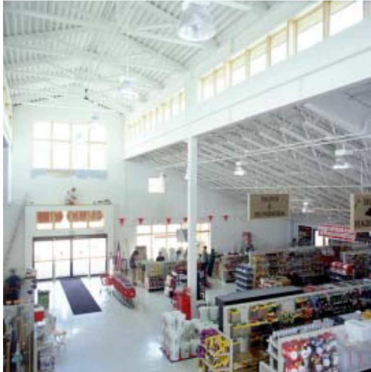
Figure 7-2 Retail area lighting with daylight only for clear sky conditions on June 5, 2000
