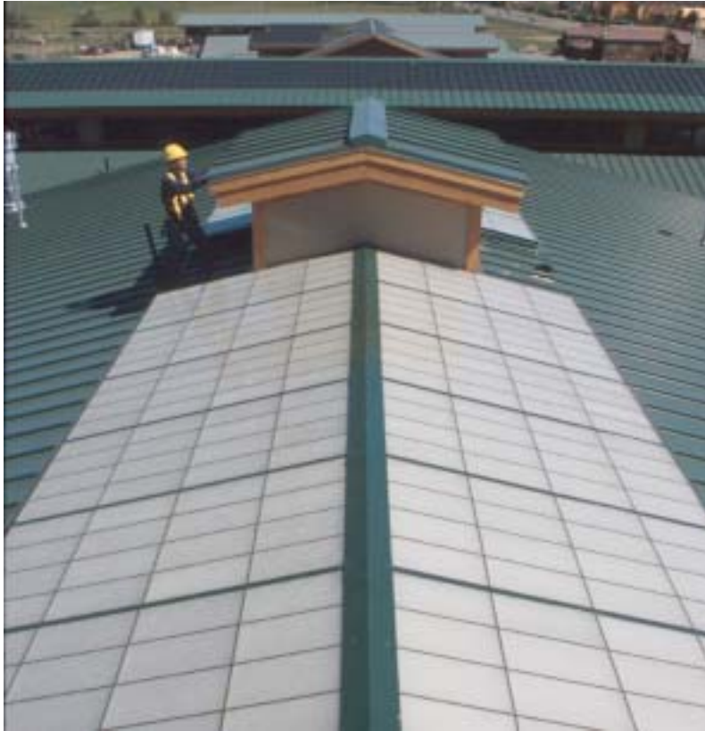
Figure 5-8 Translucent skylights in the warehouse
