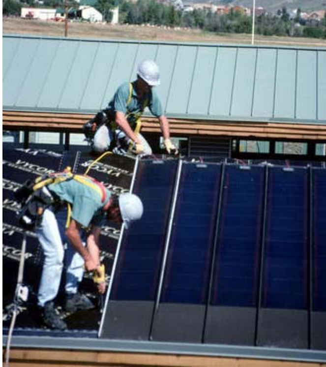
Figure 5-9 Installation of the roof-integrated PV panels
