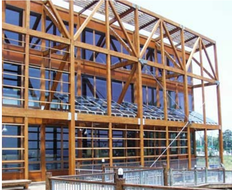
Figure 4-7 PV array and shading caused by building structure
