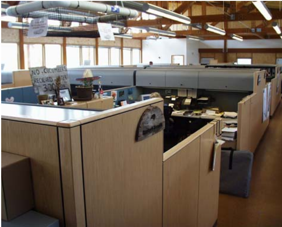
Figure 4-5 T-8 overhead lighting and task lighting on the second floor (50% direct/50% indirect)
