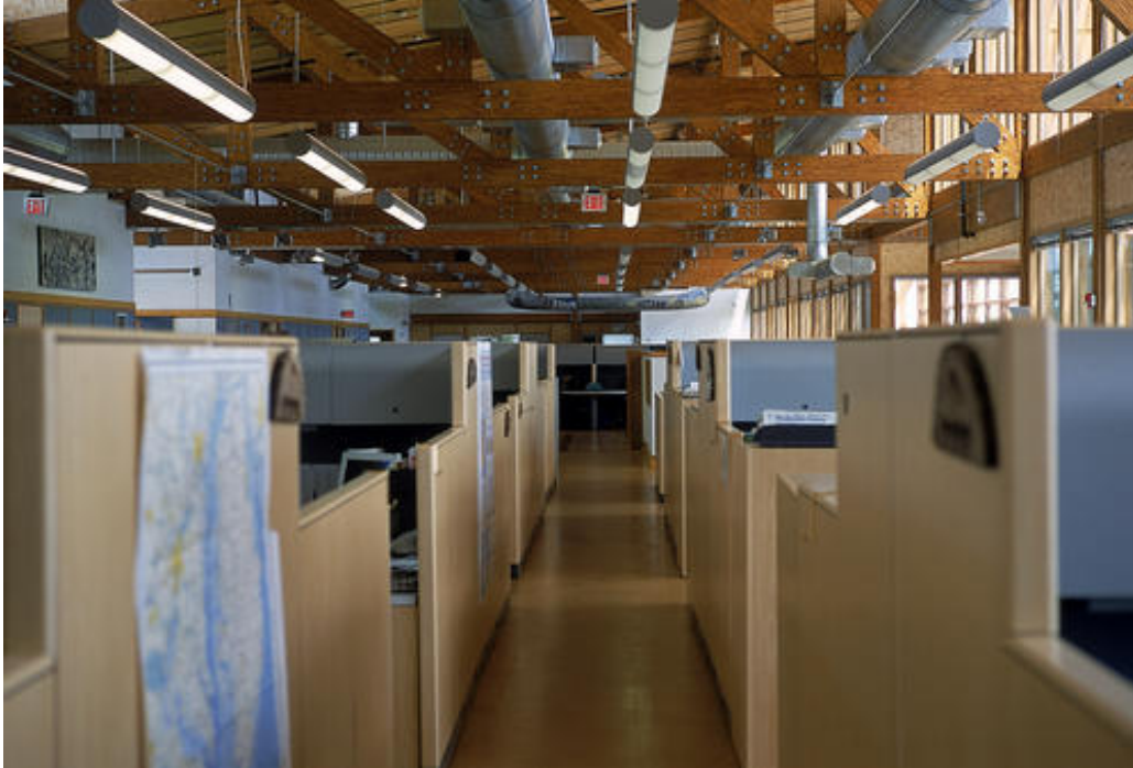
Figure 6-18 Second-floor ceiling, beams, and ducts
