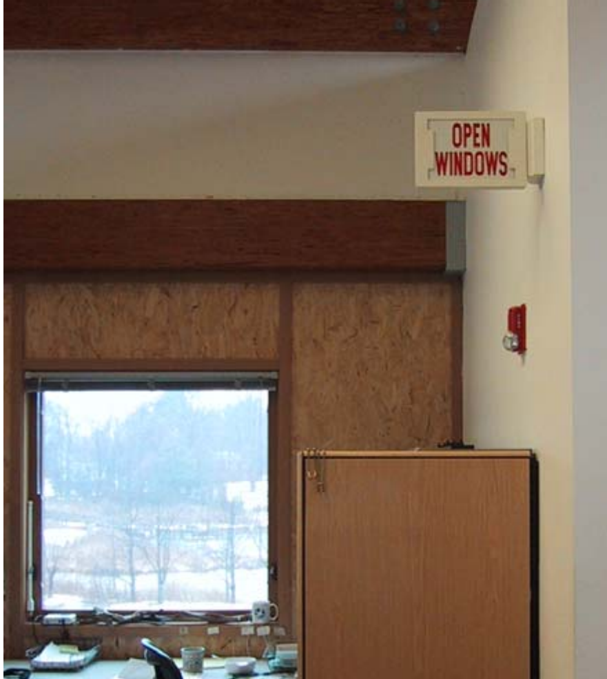
Figure 4-9 Signage directs occupants to operate windows
