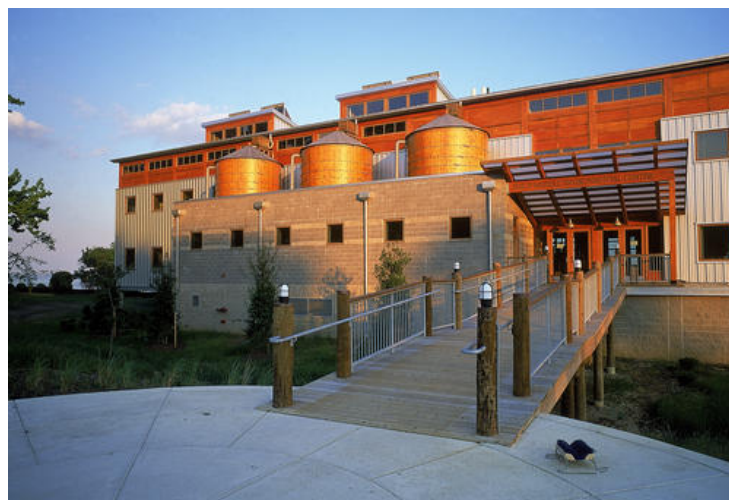
Figure 4-1 Merrill Center north entrance shows rainwater storage tanks and north clerestories
