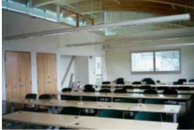
Figure D-10 Second-floor classroom showing daylighting without electric lights
