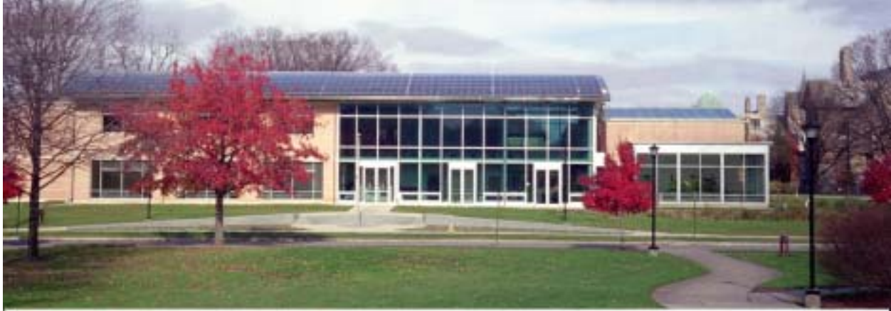
Figure 4-9 PV installation seen from south
