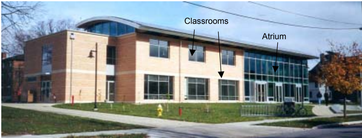
Figure 4-4 South façade of the Lewis Center
