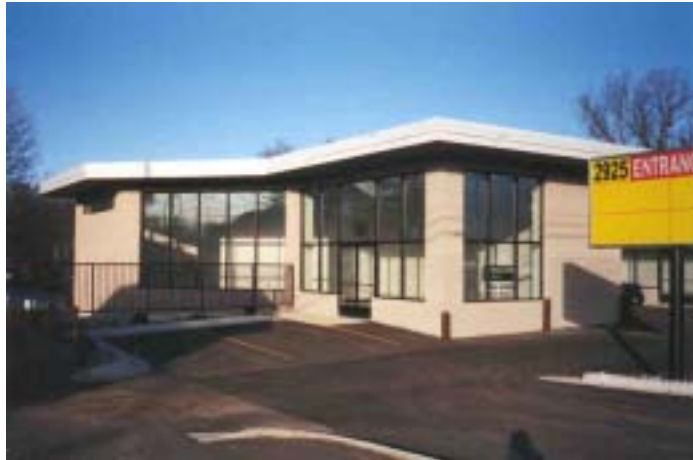
Figure 1. View of the south building from the southeast
