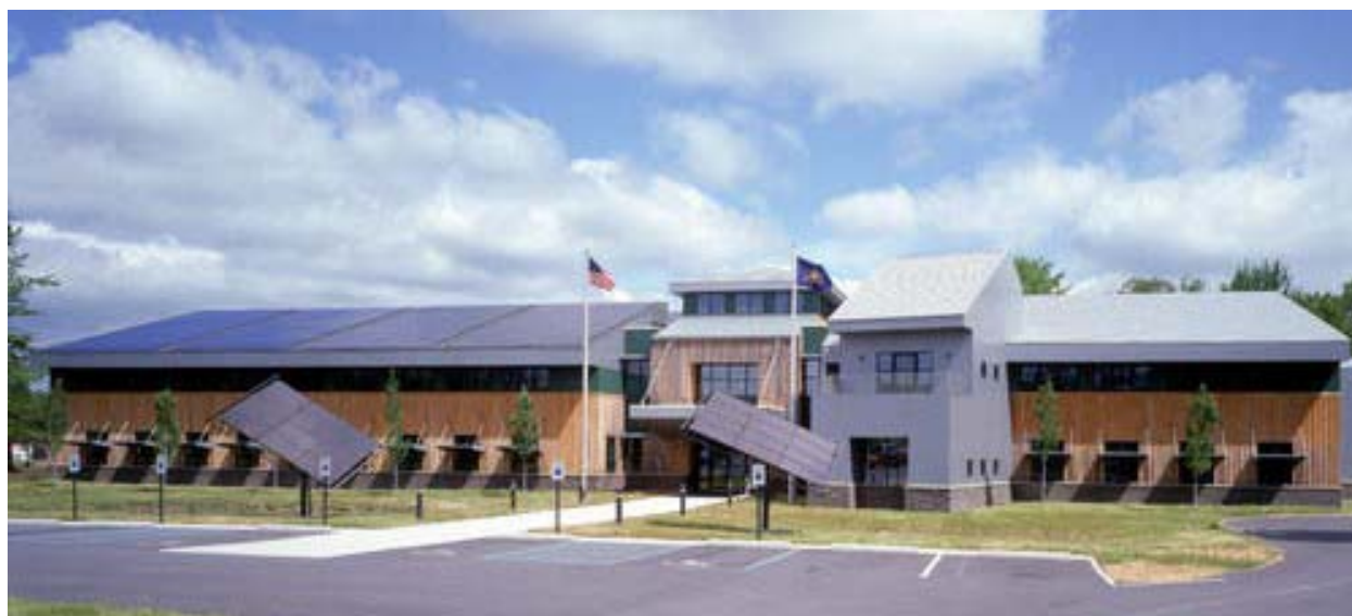
Figure 1. View of the south side of the Pennsylvania DEP Cambria office building
