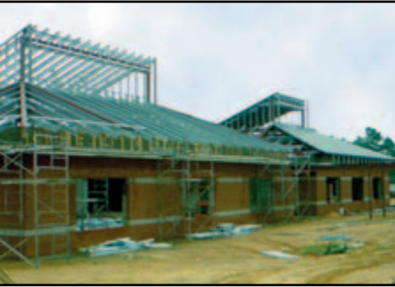
High-mass construction techniques lag the heat gain experienced during the daytime well into the evening.
