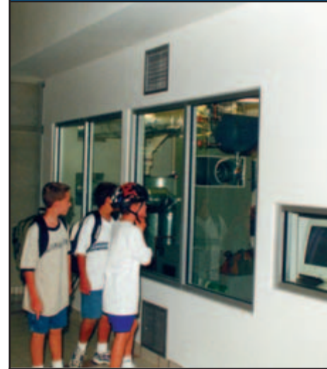
An exposed energy-efficient mechanical system can serve as an educational tool for energy conservation.
