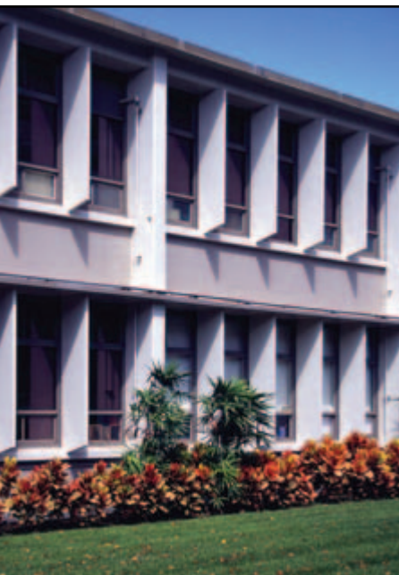
Photo: Architectural Energy Corporation At Iolani School in Honolulu, Hawaii, window overhangs provide effective shading for view windows.
