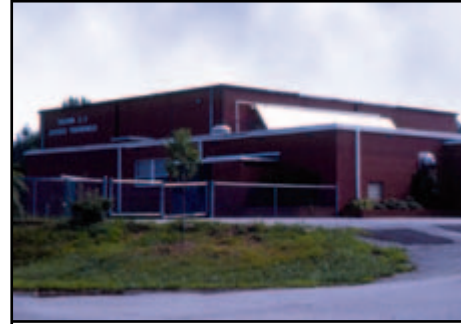
This drainback solar domestic water system was added to the school's kitchen roof area and provides most of the hot water required by the cafeteria.
