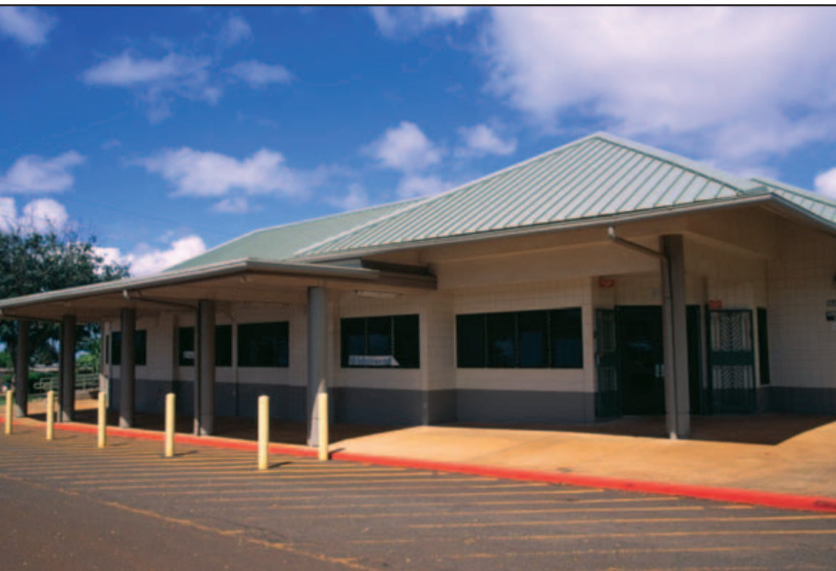
Photo: Architectural Energy Corporation Energy-efficient exterior walls, light-colored roof finishes, and window shading overhangs are among the high performance building shell elements used at Pearl Ridge Elementary School on Oahu.
