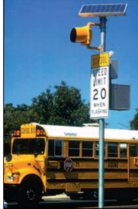
Photo: Glen Bair, by State of Texas Energy Conservation Office
