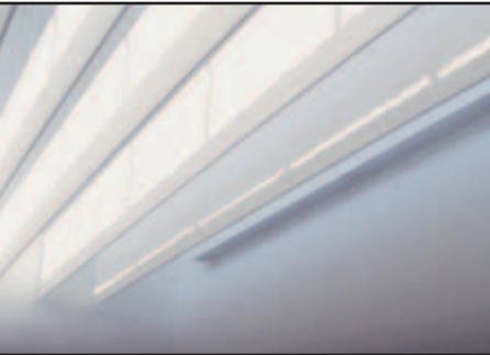
Translucent baffles block direct beam radiation and diffuse the sunlight throughout the space.
