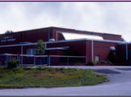
This solar domestic water system was added to the school's kitchen roof area and provides most of the hot water required by the cafeteria.
