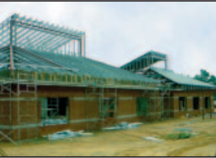
High-mass construction techniques, incorporating a brick-block cavity wall, lag the heat gain experienced during the daytime well into the evening.
