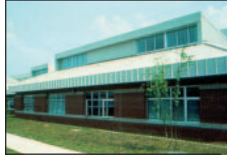
South-facing roof monitors and windows provide natural light in the classrooms.
