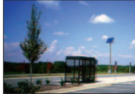
These stand-alone photovoltaic systems power parking lights.
