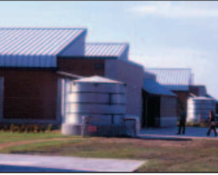
Roy Lee Walker Elementary School, in McKinney, TX, collects 700,000 gallons of rainwater each year.
