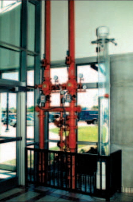
A water gauge that measures the rainwater collection tank level helps demonstrate the value of water to students.
