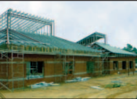
High-mass construction techniques, incorporating a brick-block cavity wall, lag the heat gain experienced during the daytime well into the evening.
