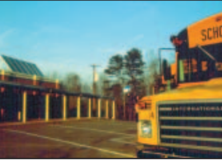
Photovoltaic systems in schools provide substantial energy savings and are educational tools.
