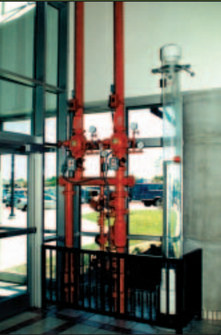
A water gauge that measures the rainwater collection tank level helps demonstrate the value of water to students.
