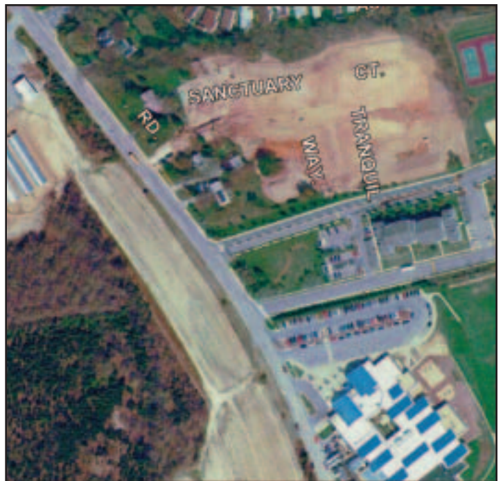
Photo: Howard County Department of Public Works
