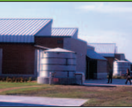
Using this cistern, the Roy Lee Walker Elementary School, in McKinney, TX, harvests rainwater.
