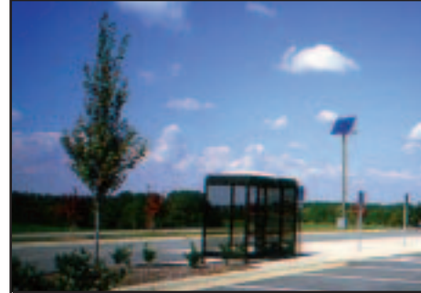
These stand-alone photovoltaic systems power parking lights.
