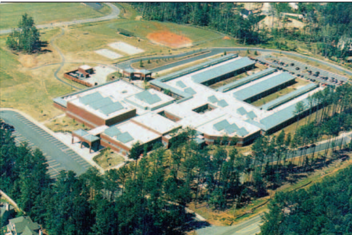
Durant Road Middle School in Raleigh, NC, is oriented on an east-west axis to maximize solar access.
