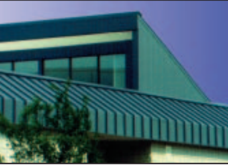
Clear double glazing has to be used to optimize solar access. Overhangs block excessive radiation in the warmer months.
