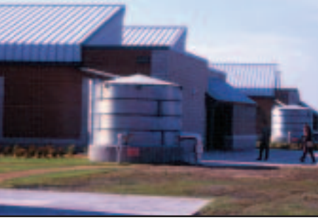
Using this cistern, the Roy Lee Walker Elementary School in McKinney, TX, harvests rainwater.
