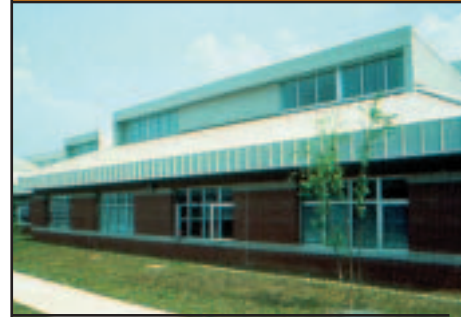
South-facing roof monitors and windows provide natural light in the classrooms.
