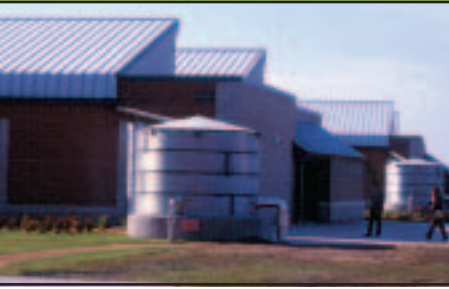
Roy Lee Walker Elementary School, in McKinney, TX, collects 700,000 gallons of rainwater each year.
