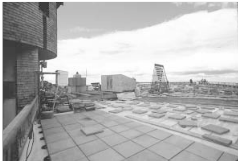
When the roof membrane was replaced on the Mount Washington Visitor Center in New Hampshire, the Styrofoam ® insulation was able to be reused because it was a protected-membrane roof.
