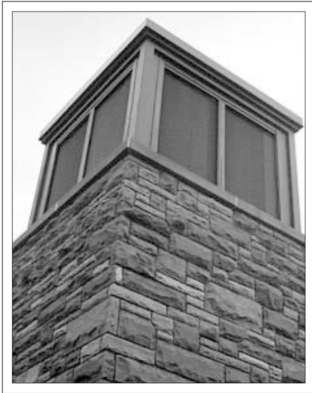
Passive down-draft cool towers at the Visitor Center in Zion National Park (in Springdale, Utah) help bring temperatures down by cooling hot air with water at the top of the tower. This cooled air then falls into the building and onto the patio.
