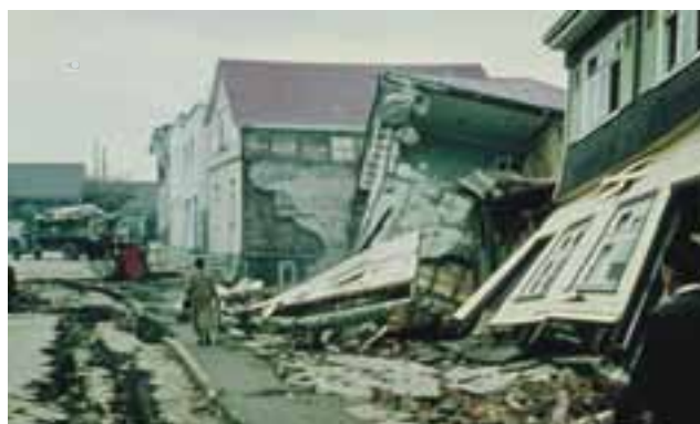
Cracked street and variably damaged buildings, Valdivia.
