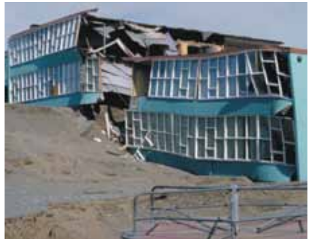
School torn by landslide, Anchorage.
