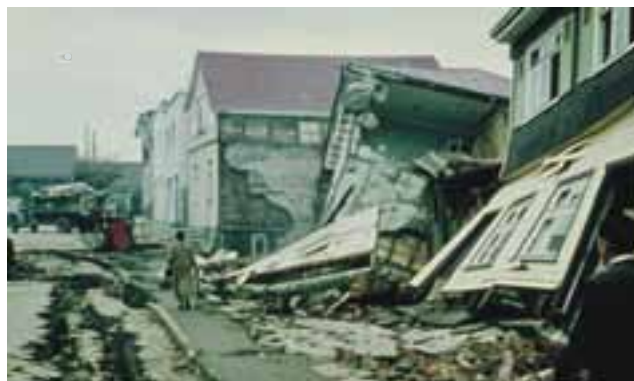
Cracked street and variably damaged buildings, Valdivia.
