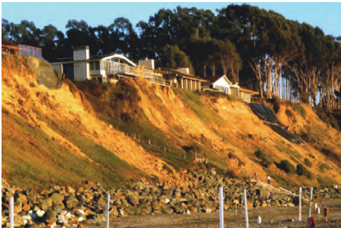
Figure 39. Shallow bluff failures that originated near the top of a moderately sloped sea cliff in northern Monterey Bay following the 1989, magnitude 6.9 Loma Prieta earthquake.
