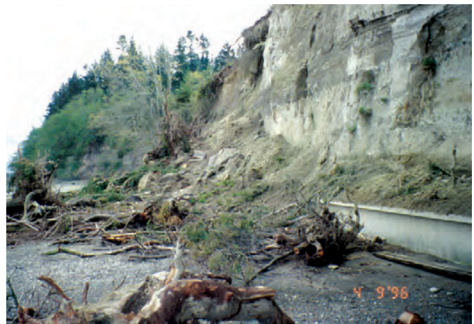
Figure 4. Failure of this steep bluff in glaciofluvial and glacial sediment in Puget Sound, Washington, occurred despite a stabilization attempt. The seawall was built to prevent toe erosion the year prior to failure of the slope.
