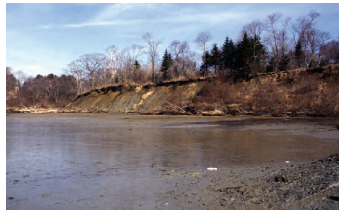
Figure 9. Eroding bluff of glacial-marine sediment, Brunswick, Maine.
