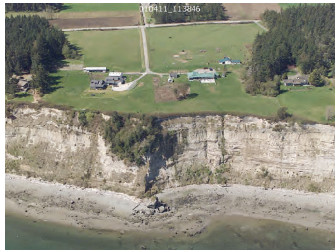
Figure 11. Offset in bluffs resulting from the presence of large glacial erratic in the nearshore. Wave action and longshore drift are from left to right. The boulder acts as a groin—on the left side the beach is relative stable, but erosion has been exacerbated on its downdrift side.
