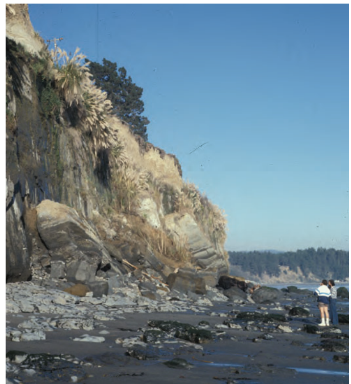
Figure 26. Block failure along joint sets accelerated by seepage in sedimentary rocks of northern Monterey Bay, California. Seepage imparts a dark shade to the cliff, visible at the left side of the photo.
