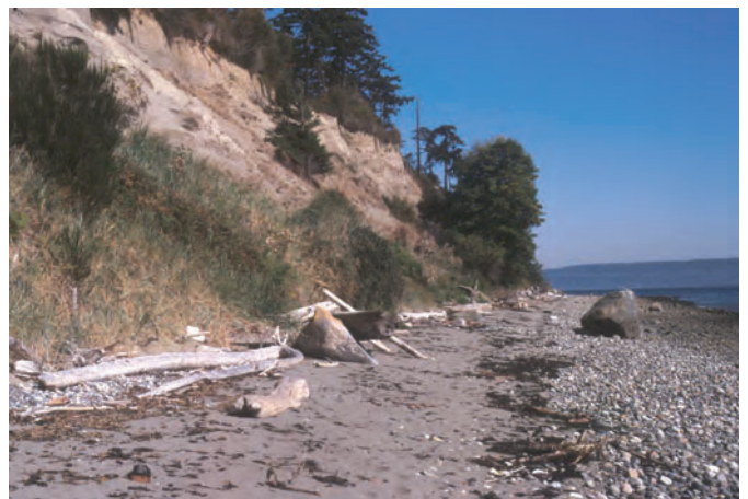
Figure 6. Typical mixed sand and gravel beach at base of high coastal bluff on Puget Sound. Berm, which consists of sandy material overlying a coarse gravel core, protects slope toe from wave action except when storm waves coincide with unusually high tides.
