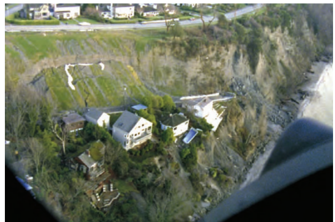
Figure 15. Homes destroyed by landsliding along Magnolia Bluff in Seattle during the winter of 1996-97. Homes had been built on a mid-slope bench formed by past erosion and landsliding.
