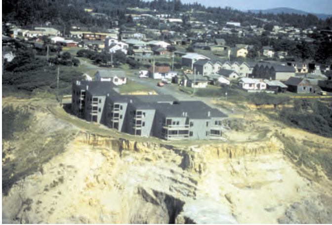
Figure 19. The condominiums built in 1981 on the remnant terrace immediately north of the Jump-Off Joe landslide in Newport. (From Sayre and Komar, 1988.)
