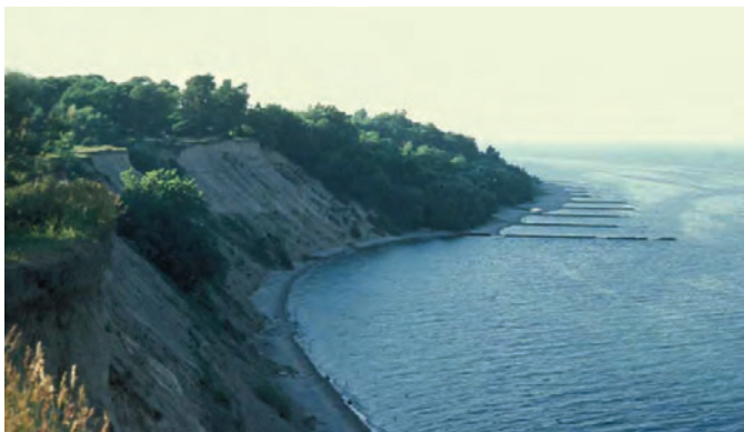
Figure 5. South of Milwaukee, Wisconsin, on Lake Michigan, groins protect the bluff in the distance, but serve to enhance erosion of the bluff in the foreground.
