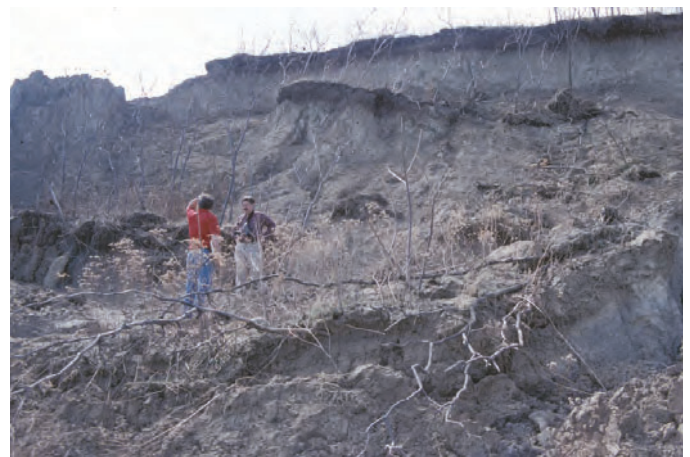
Figure 38. Slump on west shore of Lake Michigan, showing characteristic backward rotation of surface of block (above and to right of people).
