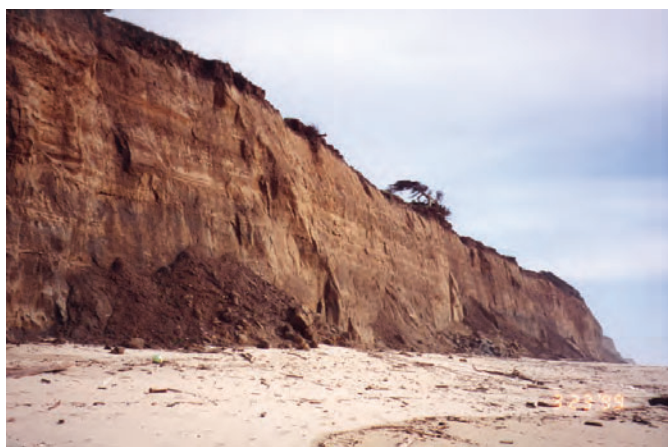
Figure 34. The relatively large failure scar on this coastal cliff (left foreground), rather than being formed by a single landslide, developed gradually as a consequence of many small block falls, the remains of which constitute the debris apron. The other debris aprons in the background formed similarly. This sea cliff in northern San Mateo County, California, retreats mainly as a consequence of small block falls.
