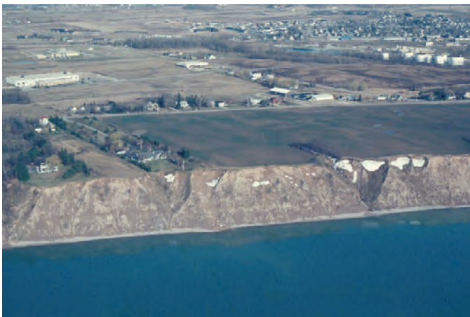
Figure 7. High (35 m) bluff of cohesive till and lake sediment on the western shore of Lake Michigan north of Milwaukee, Wisconsin.
