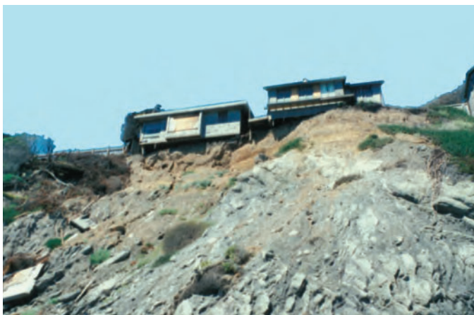
Figure 19. Ongoing cliff erosion in the Franciscan Formation of Northern California threatens cliff-top development.
