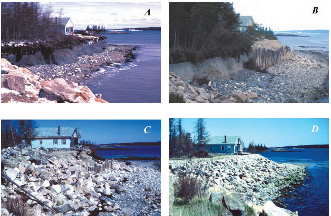
Figure 19. Typical response of homeowner to bluff erosion in Jonesport, Maine. A , 1983. B , 1985. C , 1989. D , 1993.
