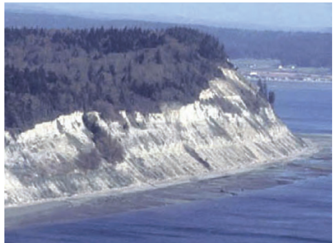
Figure 3. A moderately inclined, high bluff of sandy sediment in Puget Sound, Washington. Erosion rates are consistently at a relatively high rate here because the sediment is weak and because the exposure and orientation result in rapid longshore redistribution of sand, preventing buildup of a wide, protective beach.
