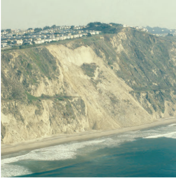
Figure 14. Seismically induced bluff failure north of Pacifica in Daly City, 1989.
