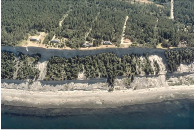
Figure 4. High bluffs near Port Townsend illustrate role of distinct stratigraphic units in defining bluff profile. Upper unit of glacial till fails in vertical slabs and does not support vegetation. Central sandier outwash unit is at angle of repose, with substantial revegetation between erosional events. Lower glacial unit is subject to wave action when storms and high tides coincide and when beach volume is reduced.
