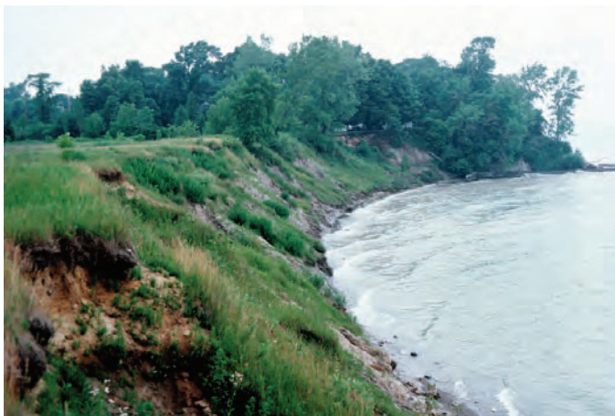
Figure 4. Low cohesive bluff (10 m) with simple profile and parallel retreat on the southeastern shore of Lake Michigan in Kenosha County, Wisconsin.
