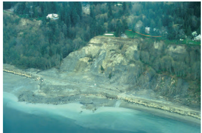
Figure 8. Large landslide north of Seattle that occurred in January 1997, following heavy rains. Note distinct mid-slope bench to the right of the landslide, marking the contact at the base of the glacial outwash. The landslide, which pushed a train into the Sound, involved a deeper failure in the underlying clay units. The toe of slope had been protected by the railroad grade at beach level for approximately 100 years and was not involved in the slide.
