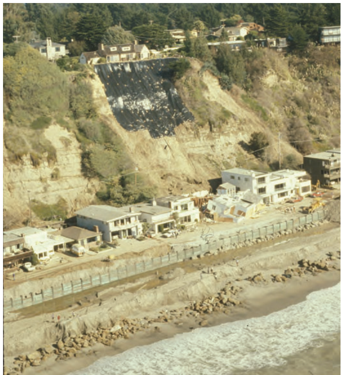
Figure 28. Shallow debris flows on this coastal cliff in Rio del Mar, California were initiated by sustained high intensity rainfall. Note the damaged houses.
