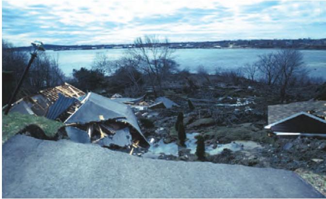
Figure 16. Landslide in glacial-marine sediment, Rockland, Maine. Two houses were lost when erosion due to the event reached more than 100 m landward from the edge of the bluff in April 1996.
