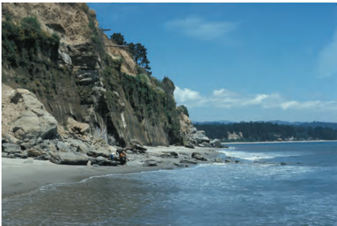
Figure 13. Episodic coastal bluff failure in Capitola, Santa Cruz County.
