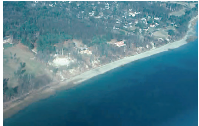
Figure 23. Aerial photo of Cumberland Foreside, Maine, with slowly retreating bluffs and valuable nearby houses.
