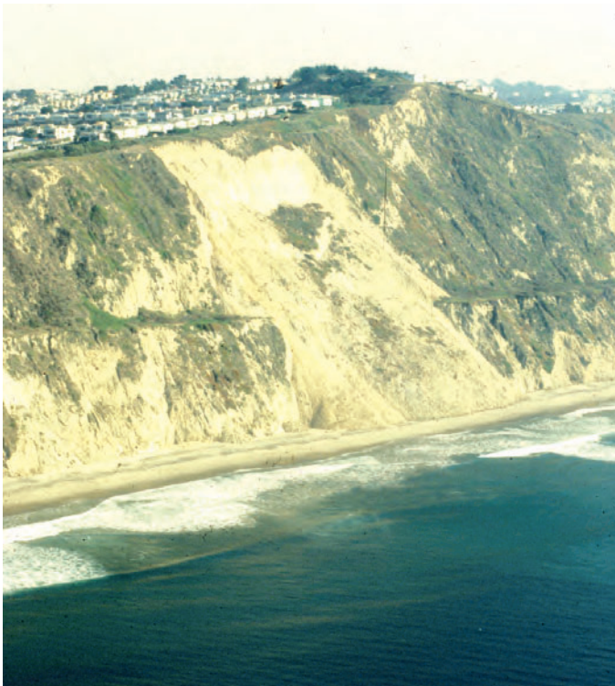
Figure 31. Large-scale coastal cliff landslide south of San Francisco, California.
