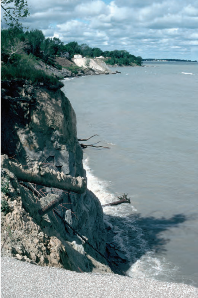
Figure 6. Low (12 m), rapidly receding bluff with complex profile that fails by slump, falls, and flows on the south shore of Lake Erie, near Cleveland, Ohio.
