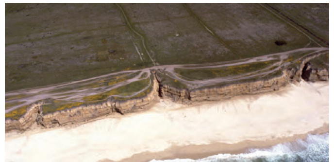
Figure 24. These large gullies at County Beach in San Mateo County, California, were carved by a combination of seepage erosion and concentrated surface runoff. Cliff is ~15 m high.
