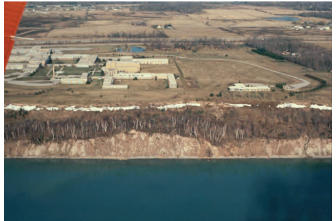
Figure 10. High (>30 m), complex bluff protected by large, deep-seated slump block that failed more than 50 years ago. Note that top of bluff is above white snow patch; slump block is below.
