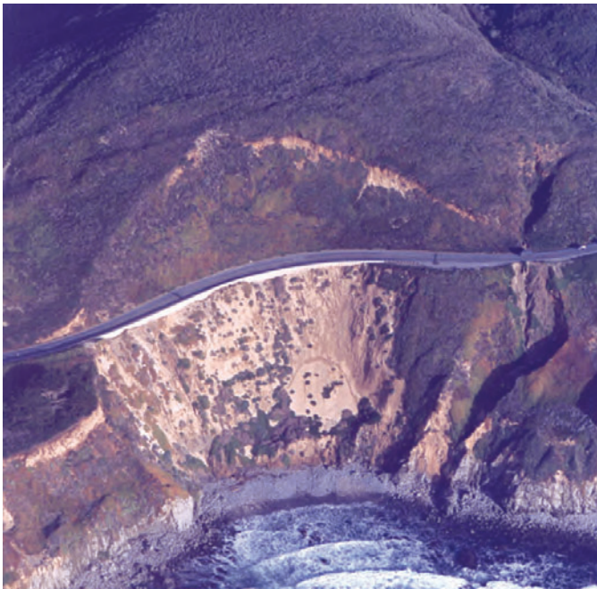
Figure 3. Movement of this large landslide on the Big Sur coast of central California is related to erosion of the coastal cliff at its base, plus other factors such as ground water. Occasional movement of large slides such as this one results in frequent damage to and associated closure of California state Highway 1, which generally follows the coast, as shown here.
