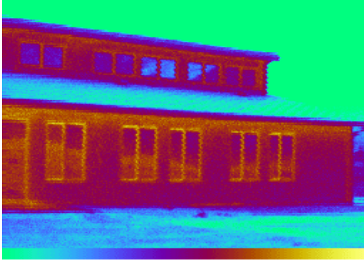
Figure 25. Infrared image of south side of house
