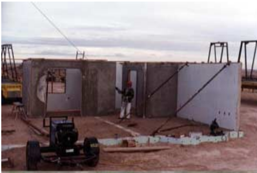
Figure 3. Pre-cast concrete walls being set up
