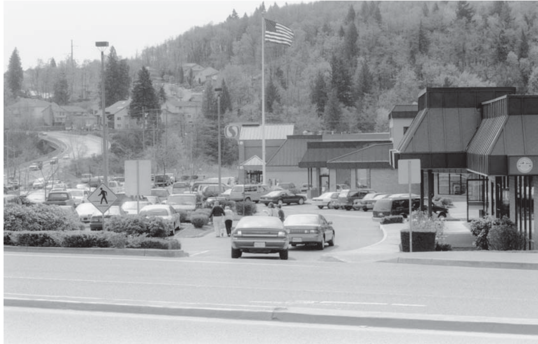
The buildings in a new Urban Business Area are clustered in a center like this one on Powell Boulevard in Gresham.
