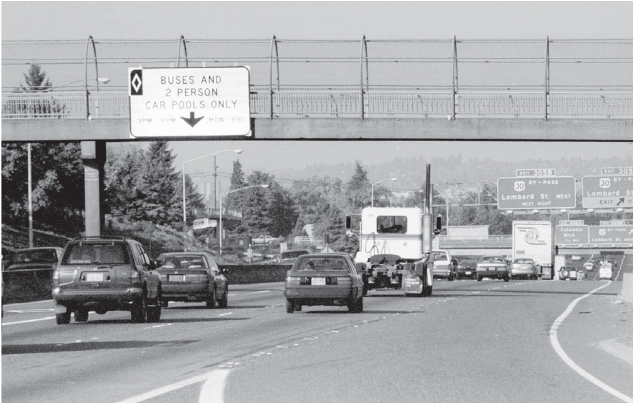
HOV facilities encourage ride sharing and help reduce congestion on Interstate 5 in Portland.
