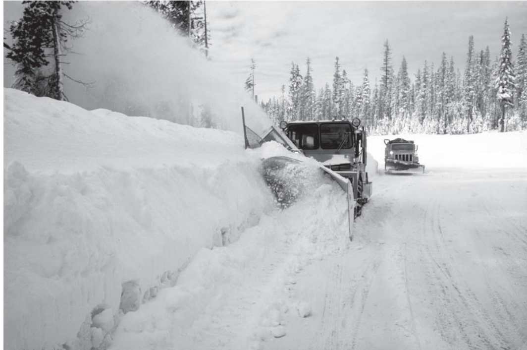
Maintenance crews respond to snow, ice, mudslides, and other weather-related conditions to keep the roads open. (Skyline Boulevard, near Mt. Bachelor)
