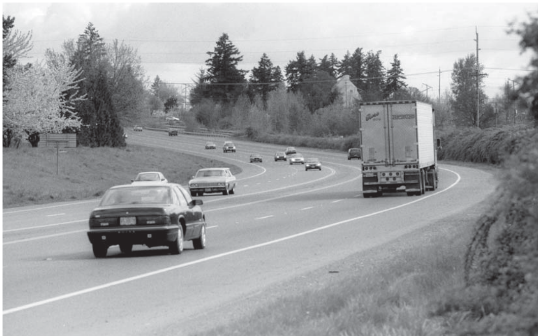
Expressways provide for high speed and high volume traffic with minimal interruption on highways like the Salem Parkway.
