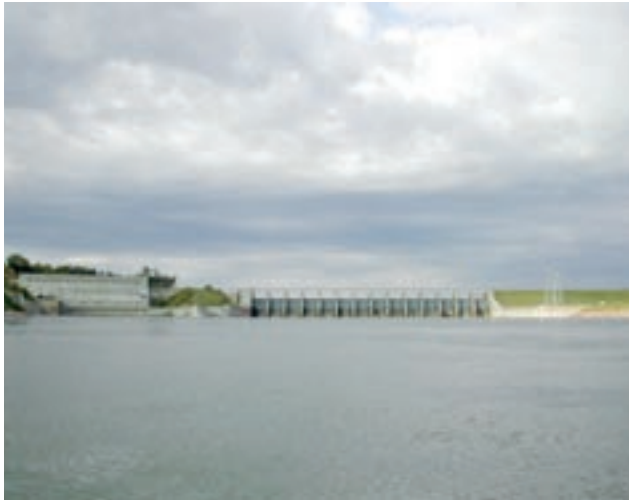
Missouri River at Gavins Point Dam (Jackson, 2003)
