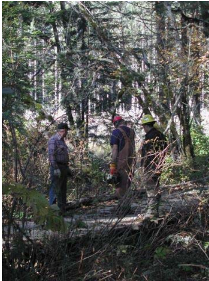
4X4 work party removing wooden bridge in an undesirable wet area
