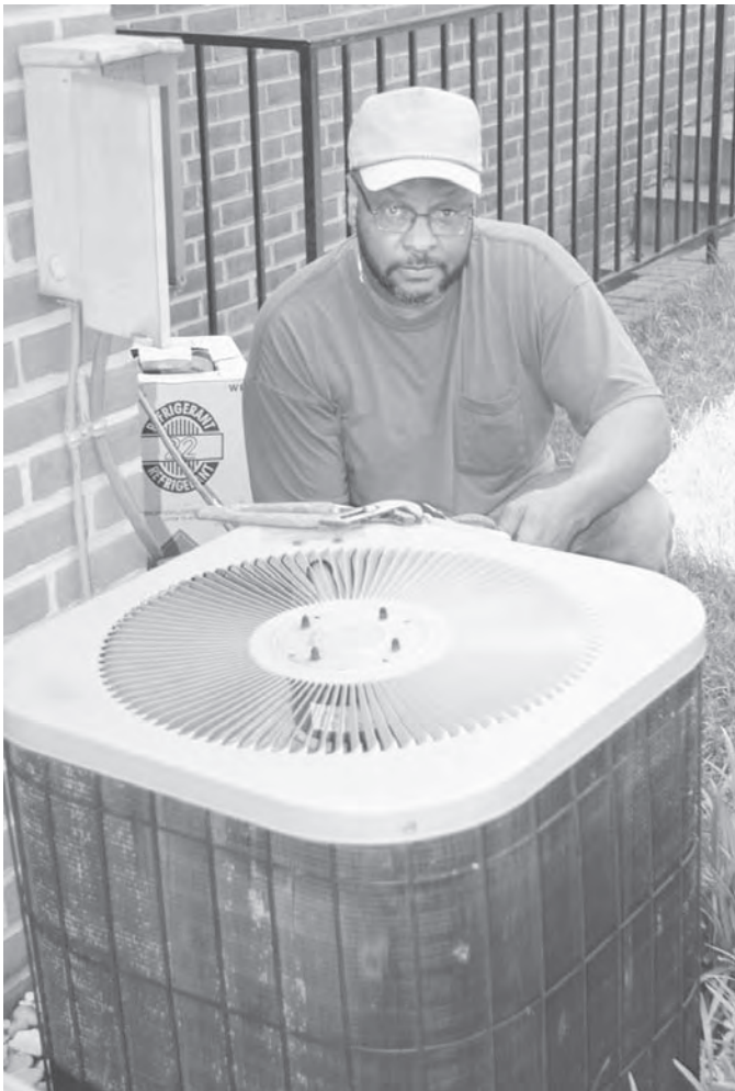
Heating and air-conditioning mechanics often work evenings and weekends, and can be on call if an emergency arises.
