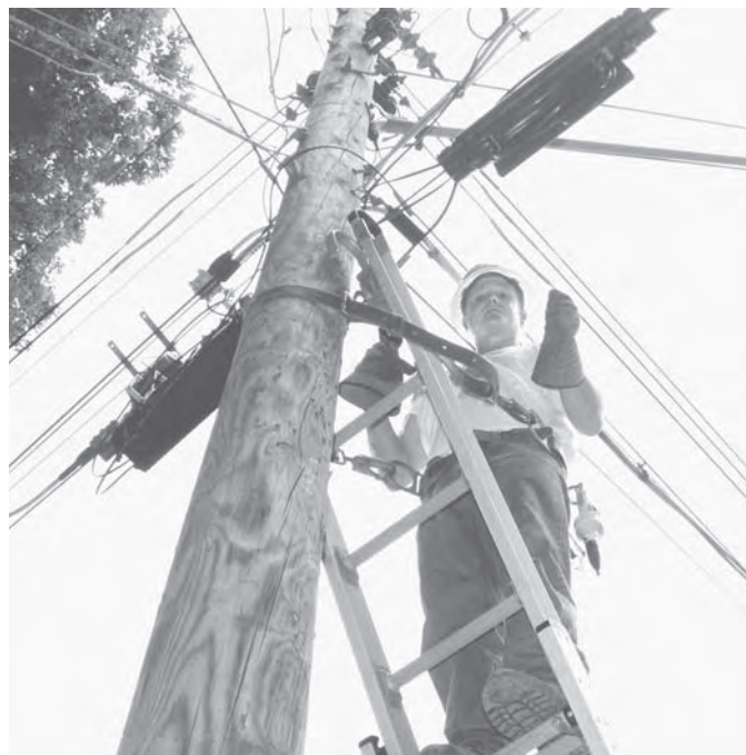
Line installers use safety equipment to prevent falls.
