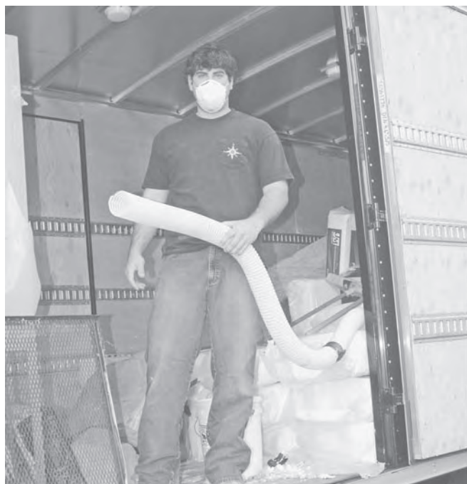
Insulation materials can irritate the eyes, skin, and respiratory system, requiring insulation workers to wear masks and other protective gear.
