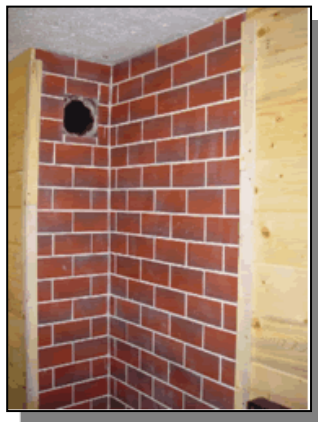
Portion of a new hearth at Jones Corral Guard Station
