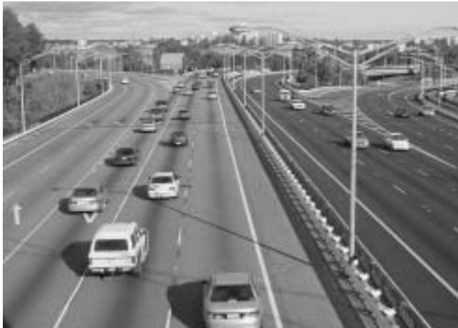
A preventive maintenance approach has helped to ensure the excellent condition of this primary highway in Perth, Australia.
