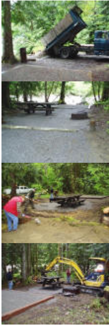
Before and after: Site rehabilitation work in progress.
