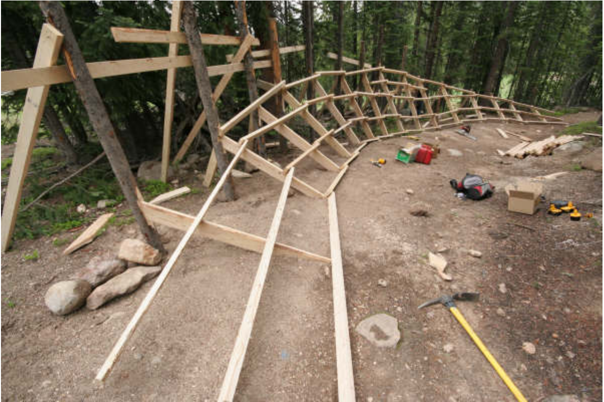
Construction of small wall ride
