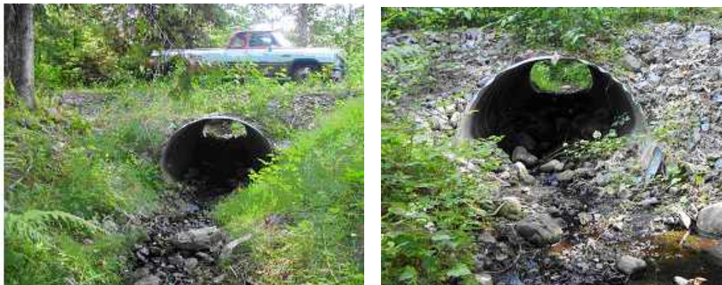
Figure 5. Road 1122000, MP 0.45; Pipe-arch three years after installation. Inlet – left; outlet – right
