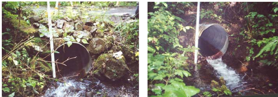
Figure 10. Fish barrier culvert Road 1122000, MP 0.51; inventoried in 2001. Inlet – left; Outlet – right
