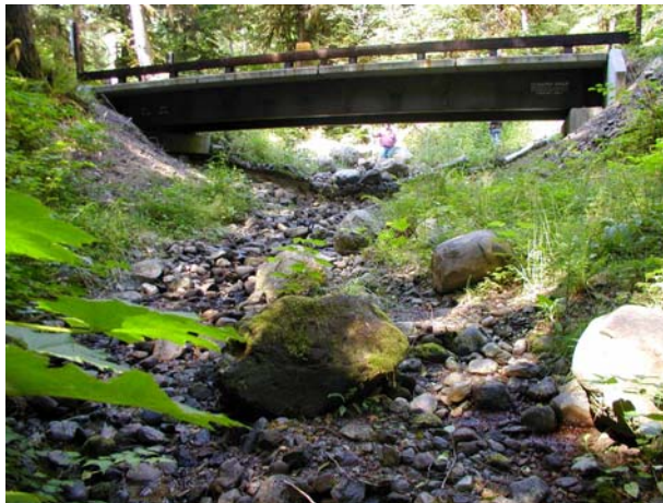
Figure 11. (Below) Bridge three years after installation
