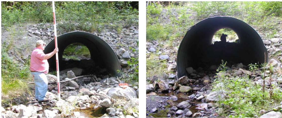
Figure 8. Road 1122000, MP 0.45; Pipe-arch three years after installation. Inlet – left; outlet – right
