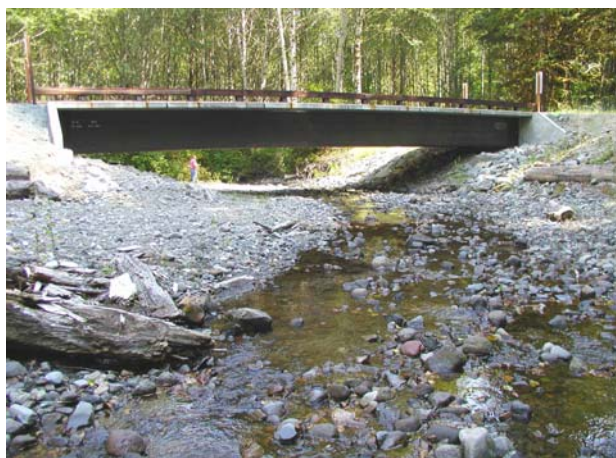
Figure 12. Bridge on Road 1122011 MP 0.18 looking downstream two years after installation.
