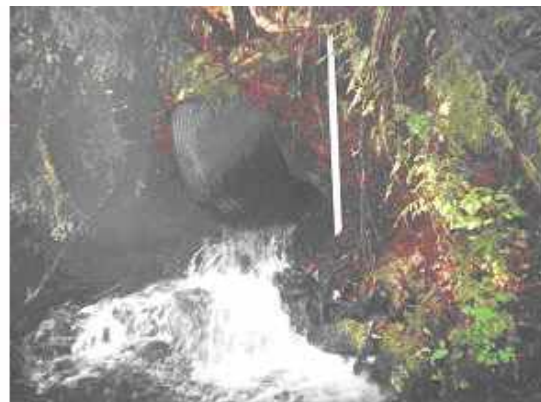
Figure 7. Fish barrier culvert Road 1122000, MP 0.49; inventoried in 2001. Inlet – left; Outlet – right
