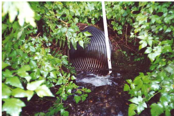
Figure 7. Fish barrier culvert Road 1122000, MP 0.49; inventoried in 2001. Inlet – left; Outlet – right
