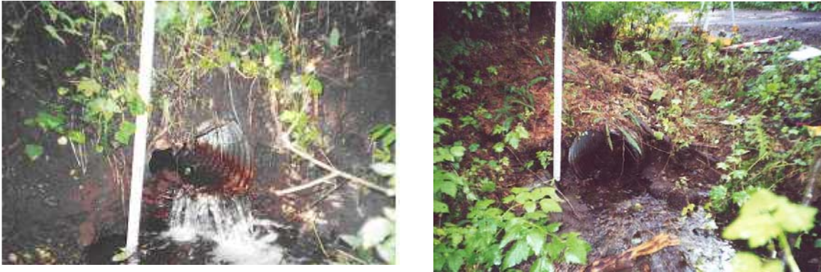
Figure 4. Photos showing fish barrier culvert Road 1122000, MP 0.45; inventoried in 2001. Inlet–left; Outlet–right
