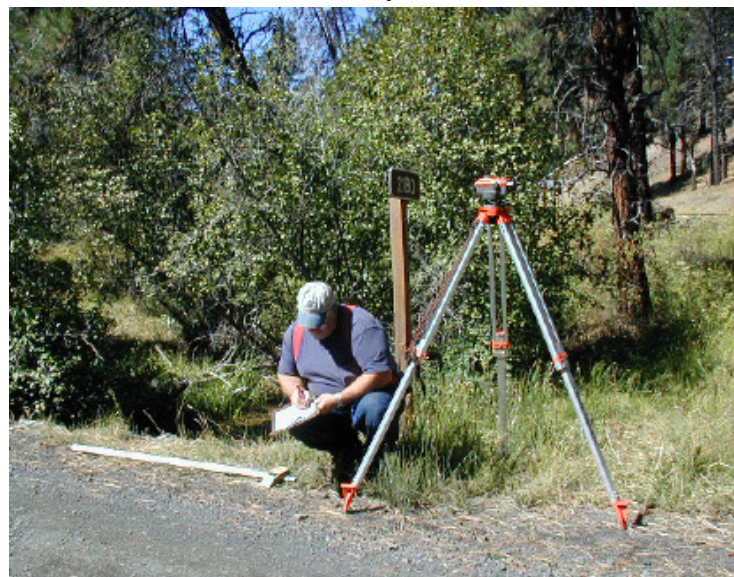
Smith at work on culvert surveys in Grant County
