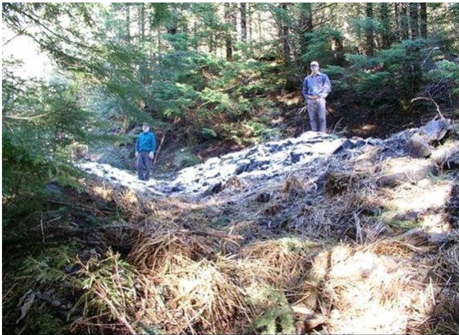
Figure II-3 Cross Drain view from outlet
