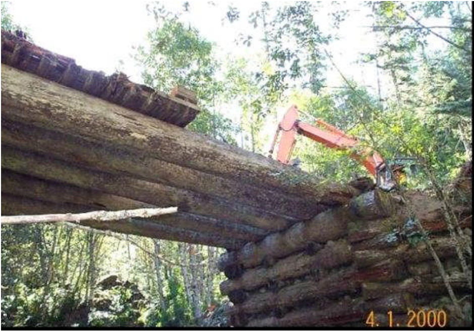
Figure II-9 Bridge Deck Removal
