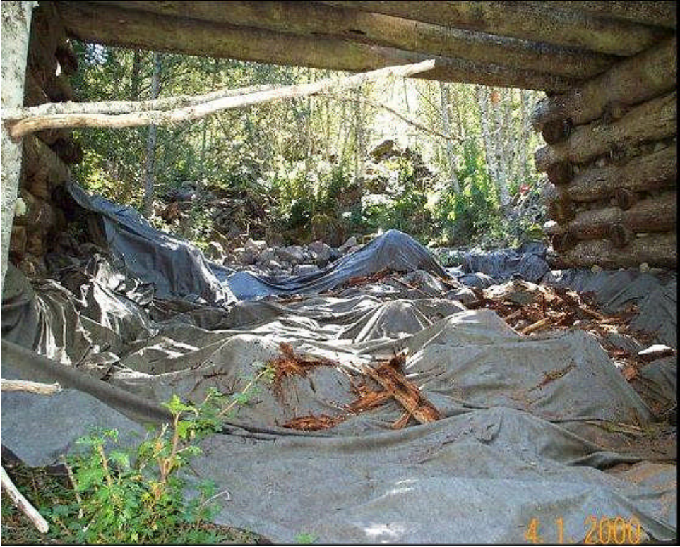
Figure II-10 Bridge Removal – Technique to keep Debris out of Stream
