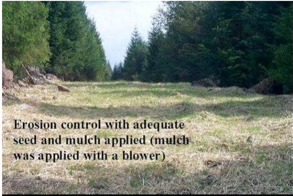
Figure II-12 Erosion Control with Seed and Mulch
