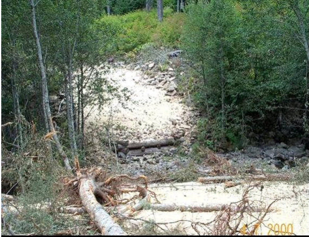
Figure II-11 Finished Bridge Decommissioning
