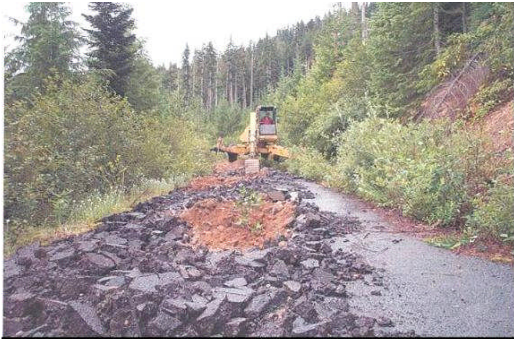
Figure II-1 Decommissioned Road Surface
