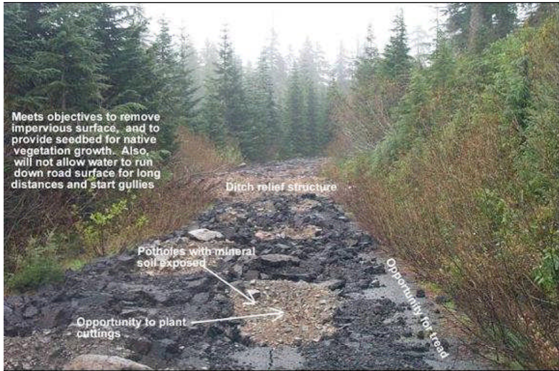
Figure II-4 Decommissioned Road Surface with Objectives Labeled
