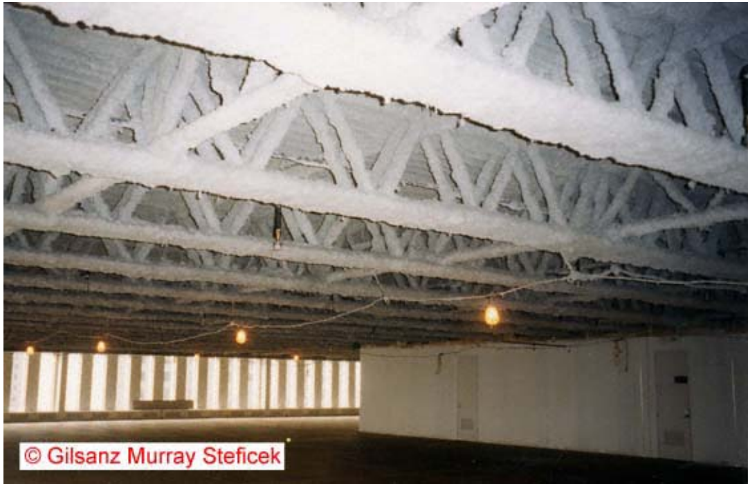
Figure 1–8. Photograph of insulated WTC trusses.
