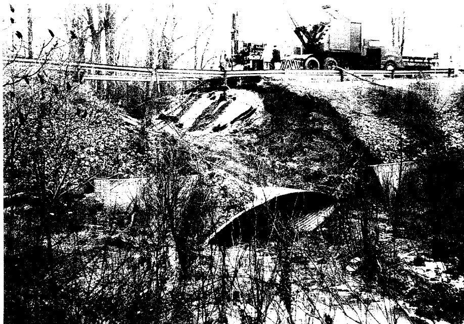
Figure 1.1 Culvert failures may be both hazardous and costly.
