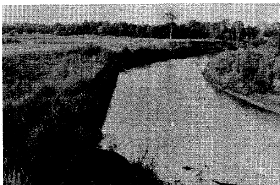
Figure 20. Timber-pile retard, at bend in channel upstream from bridge. (Washita River, Okla., Site 115.)
