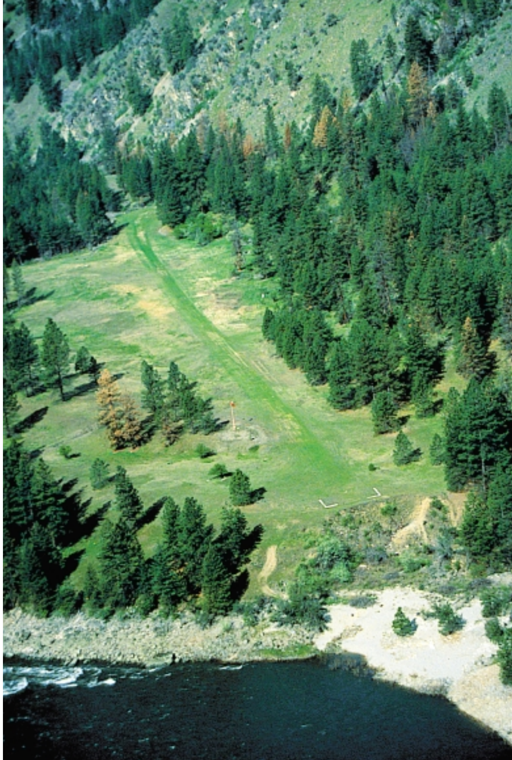
This 1,500-foot airstrip, Wilson Bar, should be used only by pilots with high performance aircraft. No go-arounds are possible, and big game animals are in the vicinity. (John Plummer photo)
