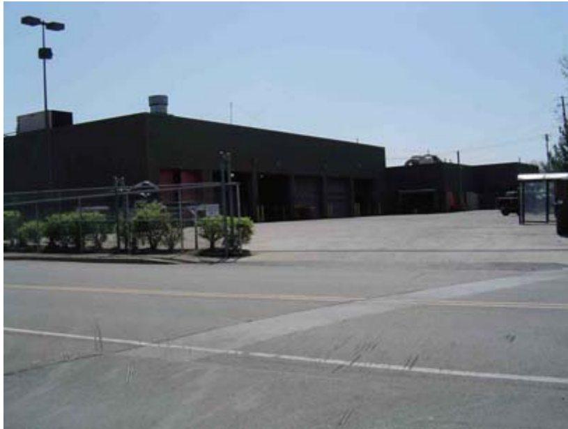
Figure 19. KAT Maintenance Facility (Source: NREL)
